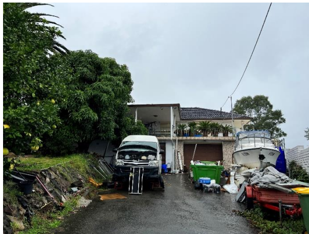
The existing dwelling to be demolished
